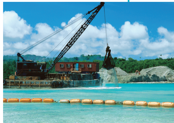
Building a new road in Babeldaob, Palau, requires dredging for gravel, a process that destroys the local marine ecosystem.
